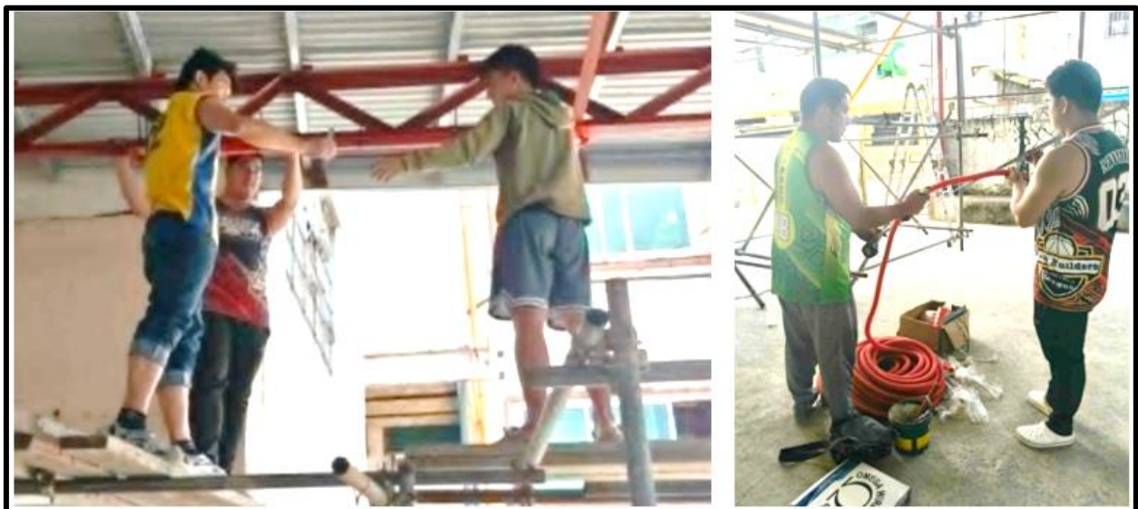
Installation of lighting fixtures at the school quadrangle, undertaken after class hours as part of the GPTA's initiative to improve campus safety, visibility, and the overall learning environment for the school community.
